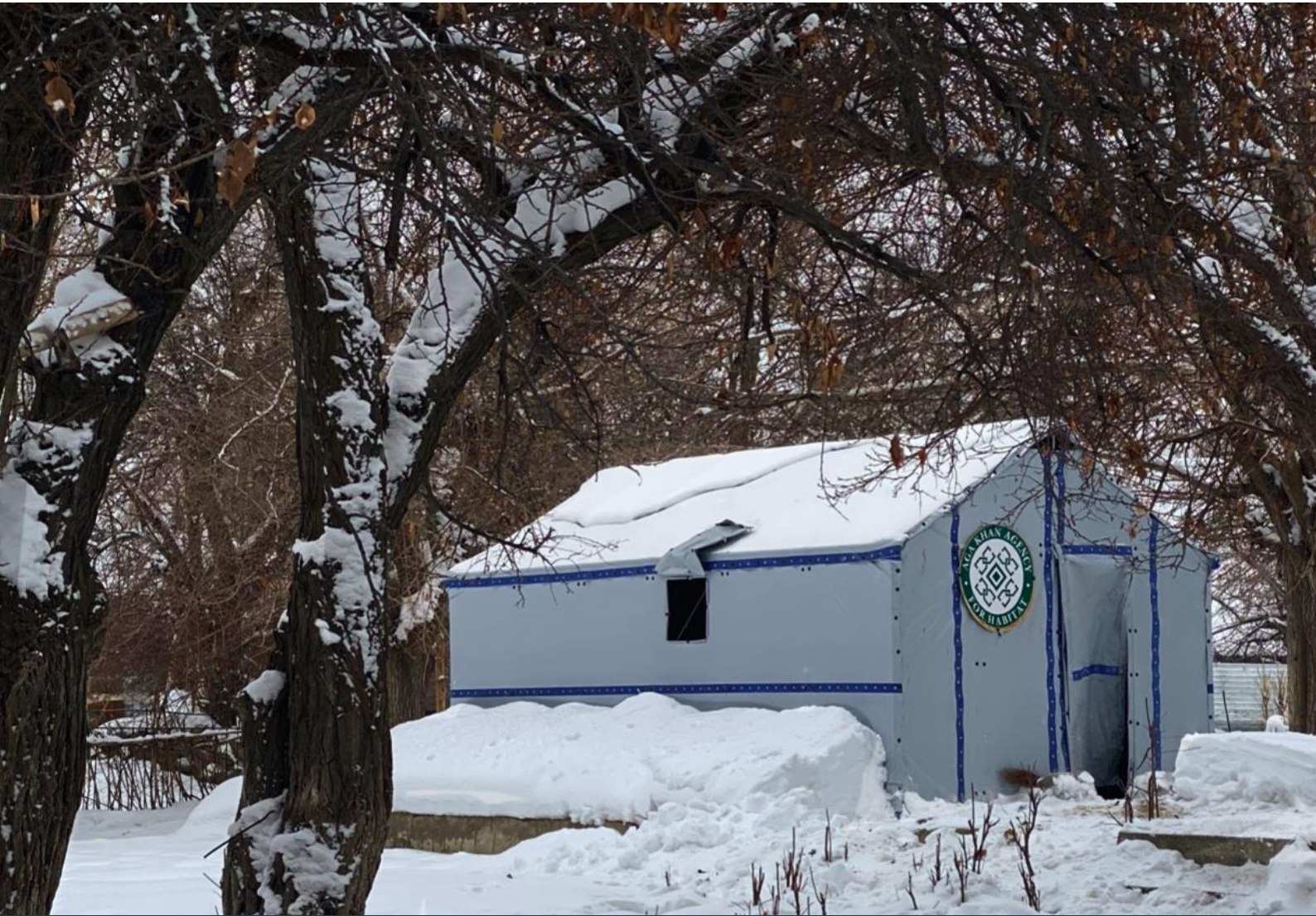
Structure Test Unit, AKAH, Tajikistan © Photo by: Sayohat Khalilova
