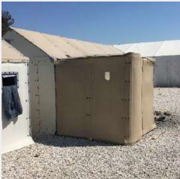
Figure 3. Reuse: Shelter extension
