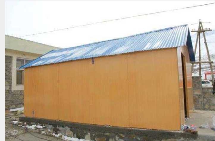
Figure 5. Reuse and Repurpose: a Structure used as vaccination point relocated in 14 places and then upgraded in a final destination as a side building of a small hospital.
