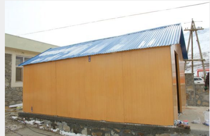
Figure 5. Reuse and Repurpose: A structure used as a vaccination point was relocated in 14 places and then upgraded to a final destination as a side building of a small hospital.
