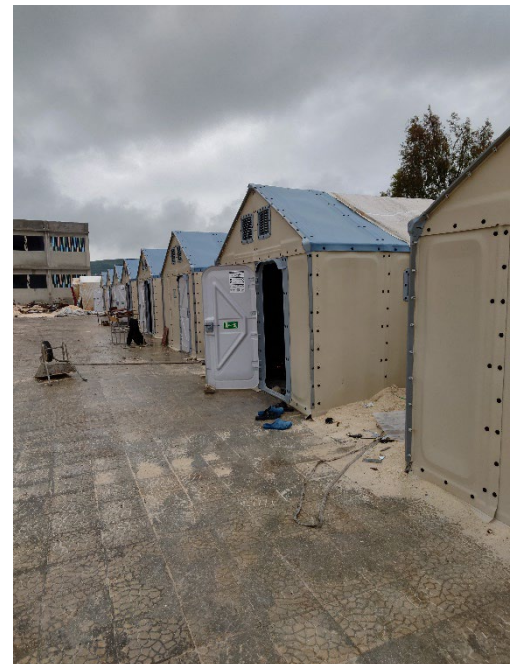
Photo 1 RHUs used as classrooms in a school under rehab
