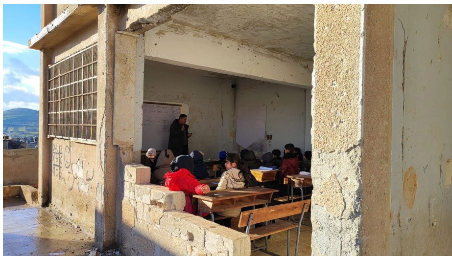
Photo 4 Lesson in a damaged classroom before installing RHUs
